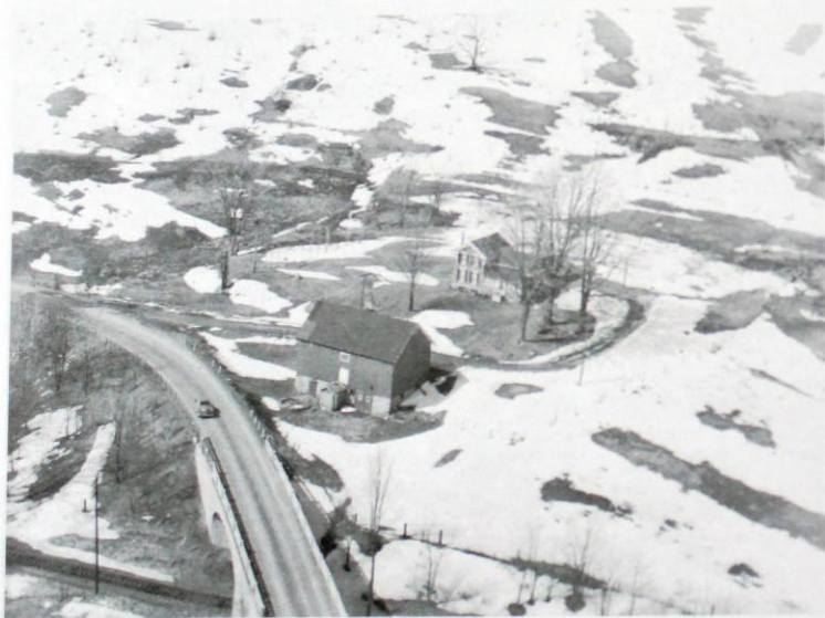
242-238 Fairchild formerly Jencks farm. Barn built in 1903, railroad bridge in 1916.
