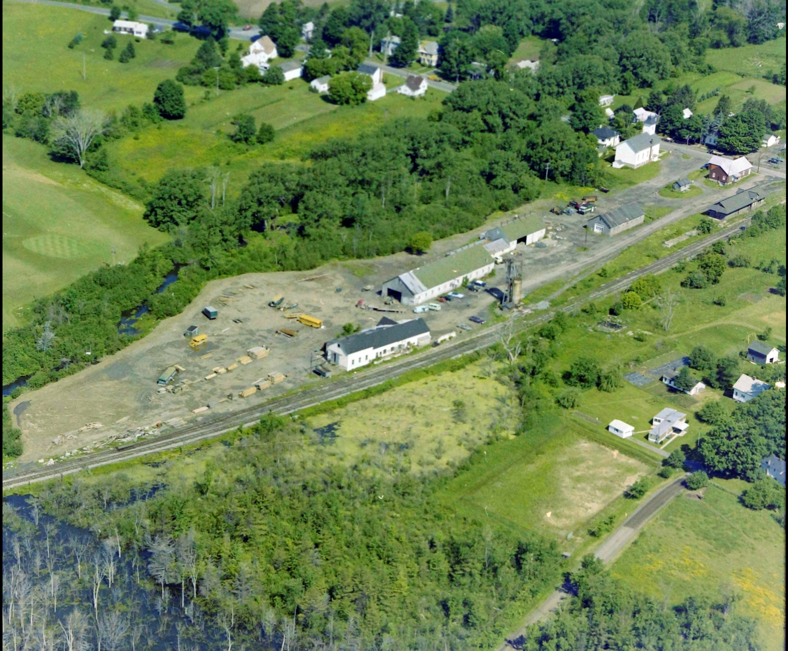
2-82 Apulia Station & the Woodford Bros Construction
