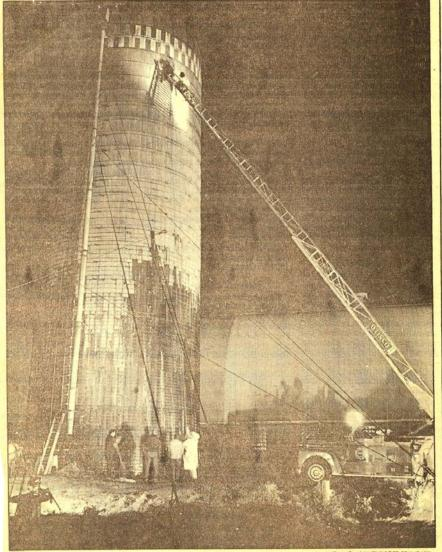
From the top of an Otisco Fire Truck ladder, Rick Woodford of Woodford Brothers Inc. straps a support cable onto a 70-foot-high silo that threatened to topple Tuesday night at the Goodrich Farms in Fabius. Fabius Fire Chief William DeHart said the concrete base of the silo had deteriorated, causing it to lean. Woodford Brothers were able to stabilize the silo - which was moving at a rate of one inch per hour - at 2:30 a.m. Wednesday. Workers spent most of Wednesday working on the structure.
