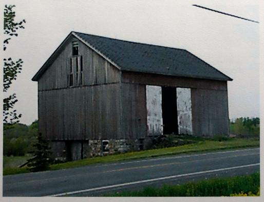
This barn was designed and built by Irving Skeele of Apulia Station. The rare Skeele design was similar to a bridge truss in that suspension of the hay mow floor was from above and therefore required no floor supports in the dairy floor below. This design is unique to our local area and allowed as much as 36 foot of clear span floor space. This feature was very rare in the late 1890 and early
